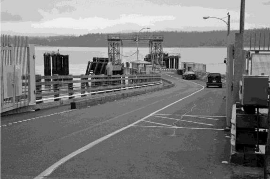
The current photograph shows the dock in 2009 with the security gate installed after 9/11, a significantly expanded passenger shelter moved to the left side, and expanded storage for ferry equipment on the right. The dock is significantly wider and a walk-on passenger walkway was added on the left side of the dock.
